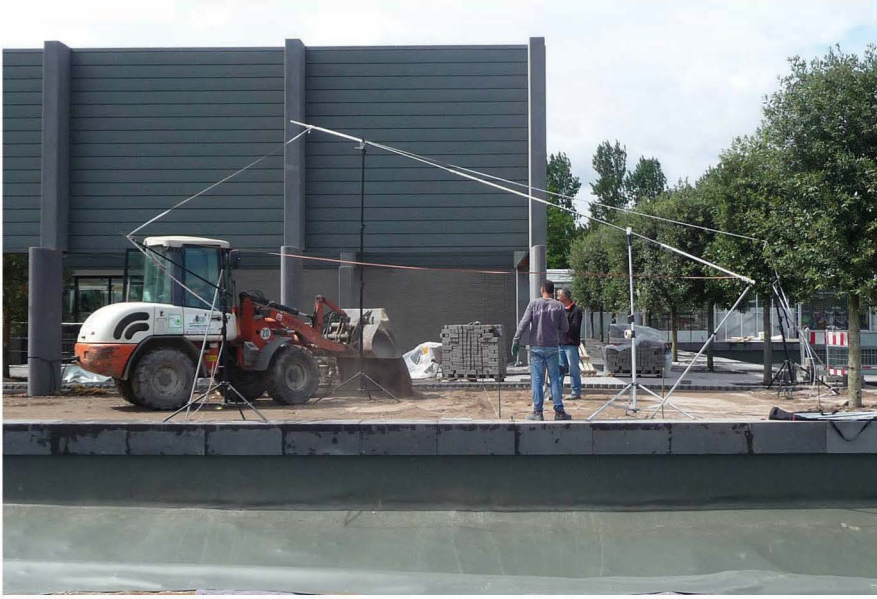
the 1 :1 simulation at the installation site
